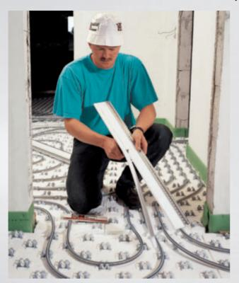
Trim the PE foam strip along the lower edge to the required height, according to the screed thickness. Mark and cut using an all-purpose blade.
