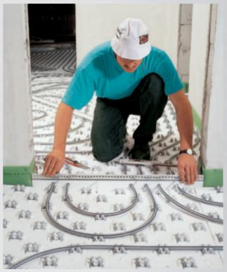
Place over the installed heating pipes and fix using dabs of mortar. Insert the plugs approx. 30 cm apart directly below the metal rail.
