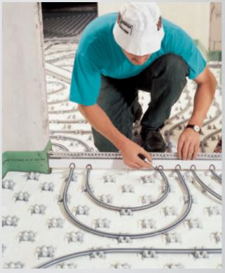
Mark the openings for the heating pipes exactly. When the profile is used between door frames, cut it to length so that it can be easily clamped between the edge strips.
