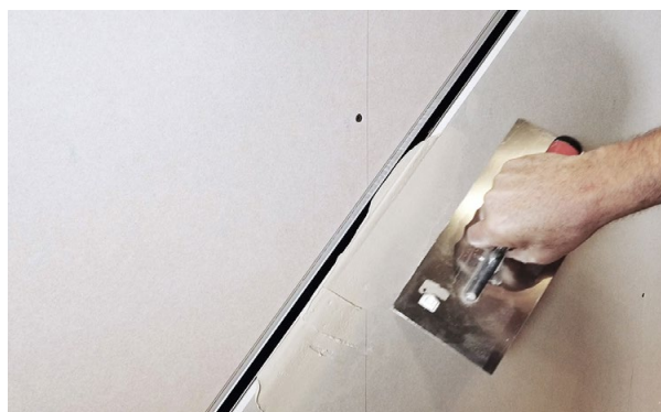
Insert and fill protective sleeve no. 6547
