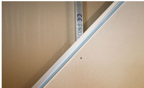
Profile fixed to the substructure and planked according to manufacturer's instructions
